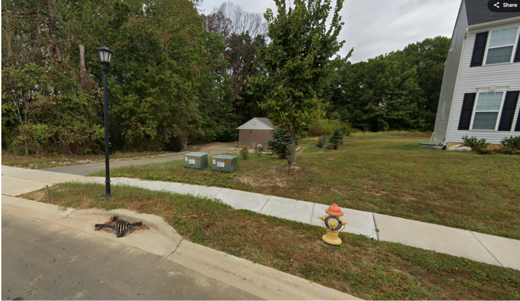
Photo 1 – North Point of Townsend Village I Pump Station adjacent to the Detention Pond next to Wiggins Mill Pond.
