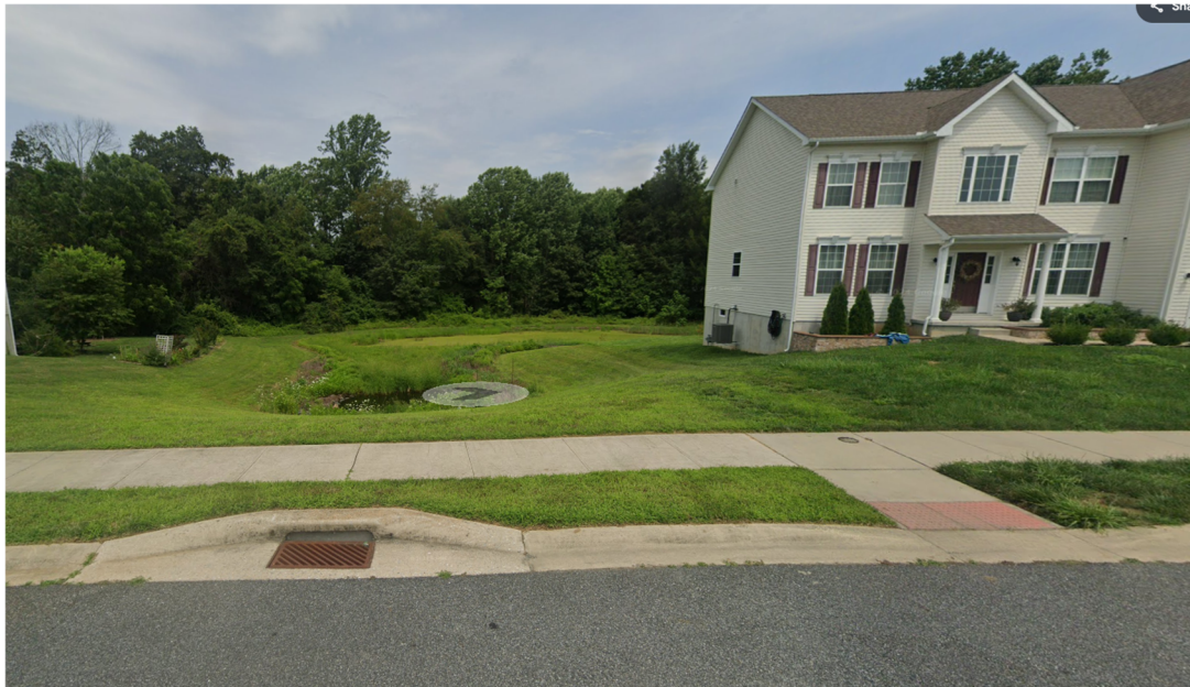
Photo No. 2 – Townsend Village II Detention Pond that discharged into the Appoquinimink River
